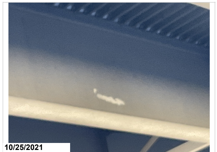
Span #2 girder #6 right side area where paint is peeling.
