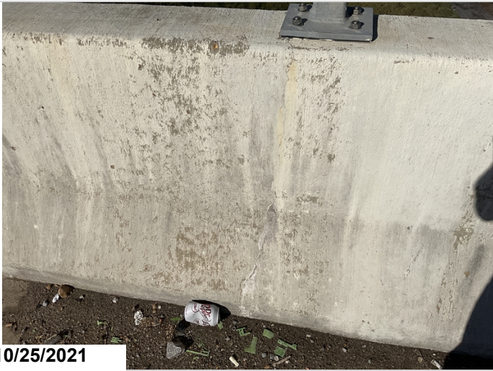
Typical bridge rail crack
