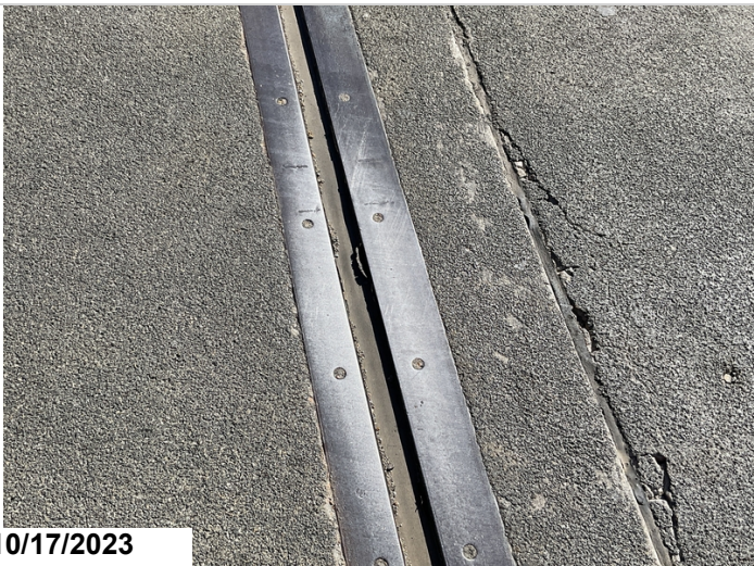
Abutment #2 joint seal right outside lane has one foot of lost adhesion
