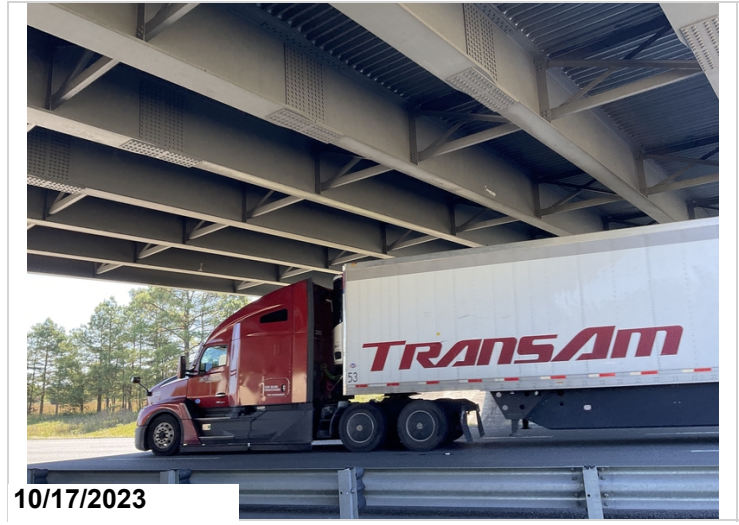
Paint peeling span #2 girders #2 and 6 right side
