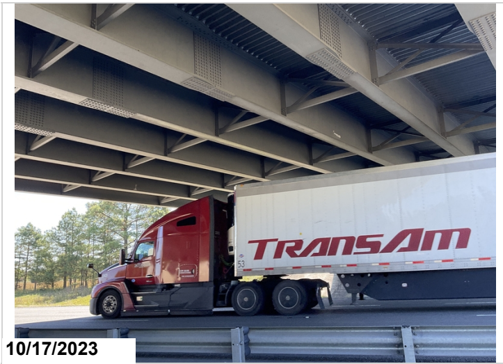
Paint peeling span #2 girders #2 and 6 right side
