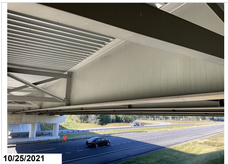
Typical interior girder condition.
