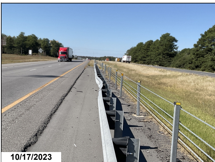
East bound lanes under bridge left lane near beginning of rail has ten feet of collision damage.
