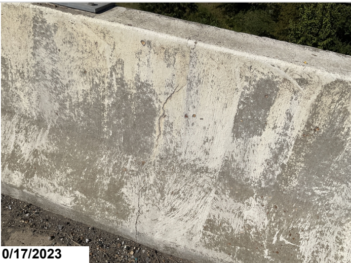
Typical vertical crack in concrete bridge rail
