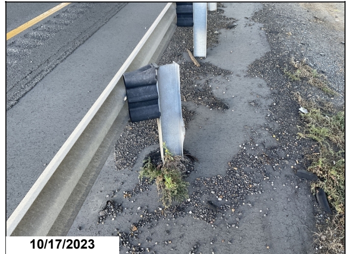
Twisted rail post west bound left rail
