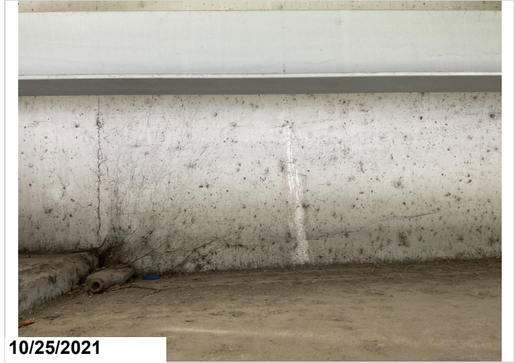
Typical abutment back wall crack
