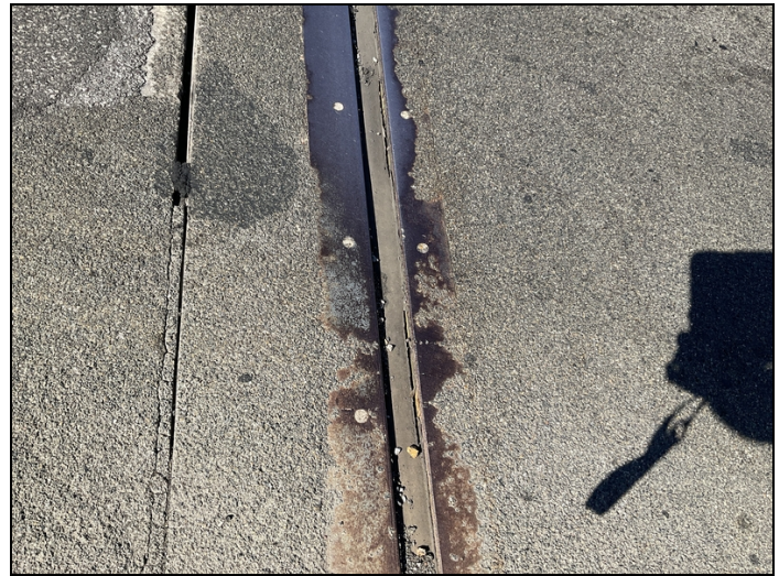
Abutment #2 joint seal has several areas of lost adhesion allowing leakage through joint.
