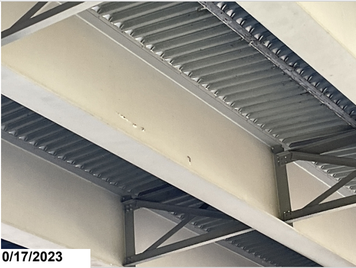
Span #2 girder #5 left side has one foot of paint beginning to peel.
