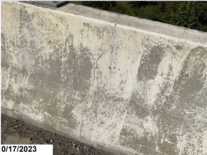
Typical vertical crack in concrete bridge rail
