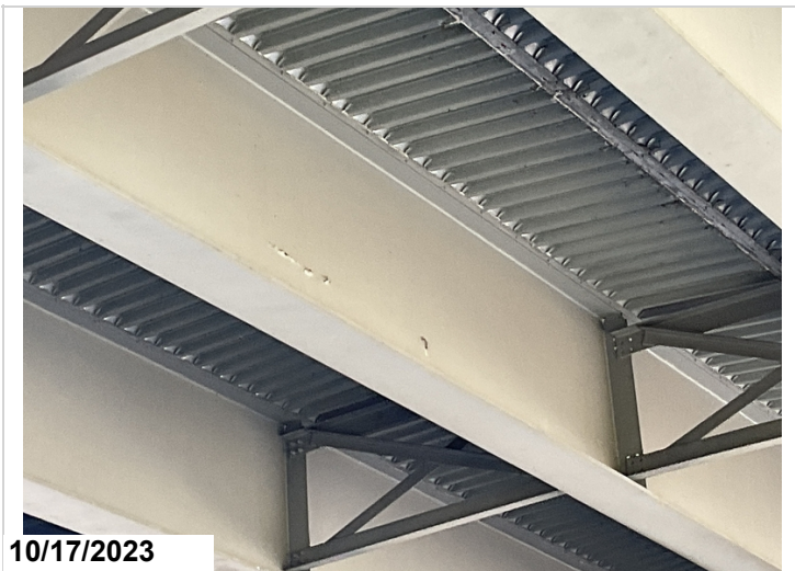
Span #2 girder #5 left side has one foot of paint beginning to peel.
