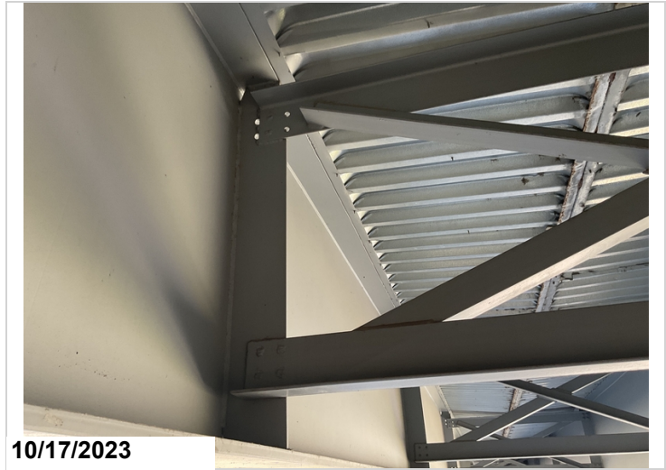
Diaphragms span #2 last 6 of them on right side are welded instead of bolted between girders #4,5.
