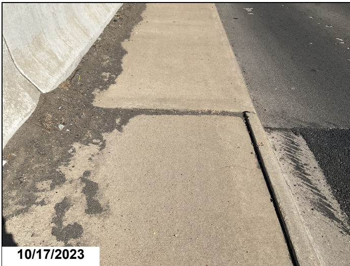
Abutment #2 right sidewalk settlement
