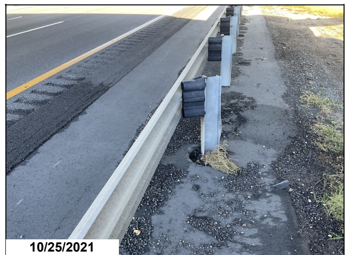
West bound roadway under bridge left lane has guardrail post twisted.
