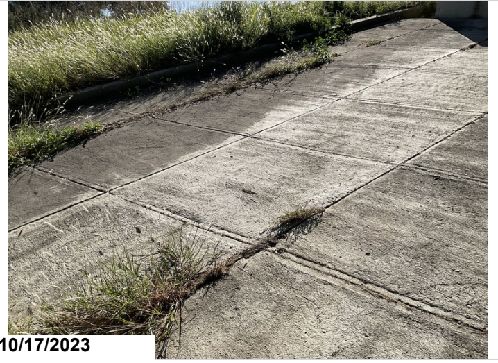
Vegetation growing left side of abutment #2 slope pavement.
