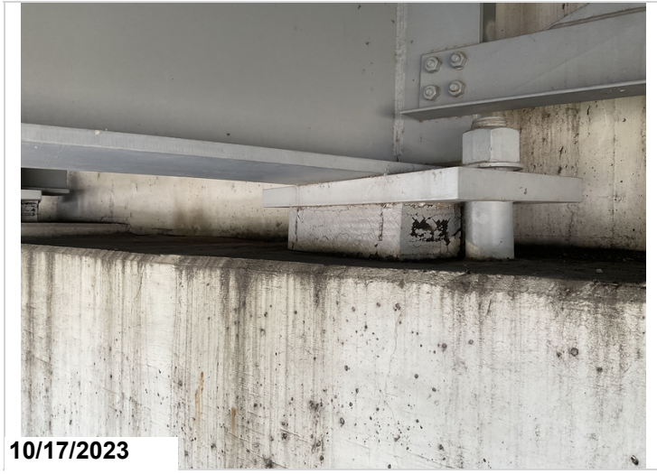
Typical abutment bearing
