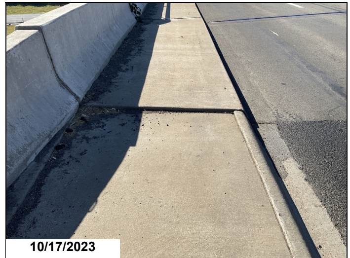
Abutment #1 left approach sidewalk has settled
