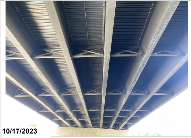
Span #1 soffit / underside of deck
