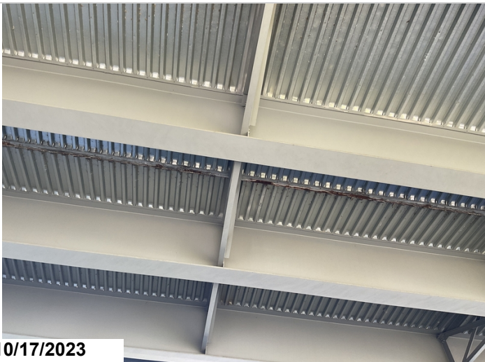
Span #2 stay in place forms beginning to corrode at centerline
