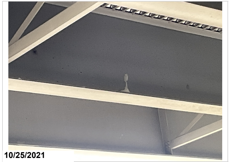
Span #2 girder #2 right side area where paint is peeling.
