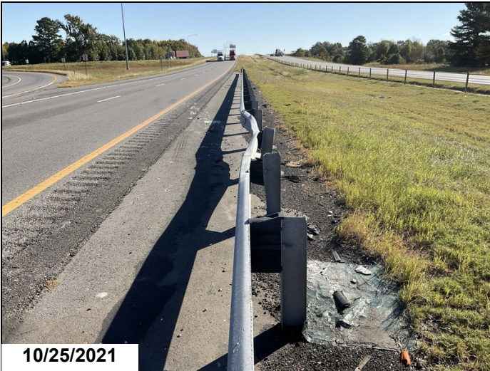
West bound roadway under bridge left lane has guardrail near beginning that has ten feet of collision damage.
