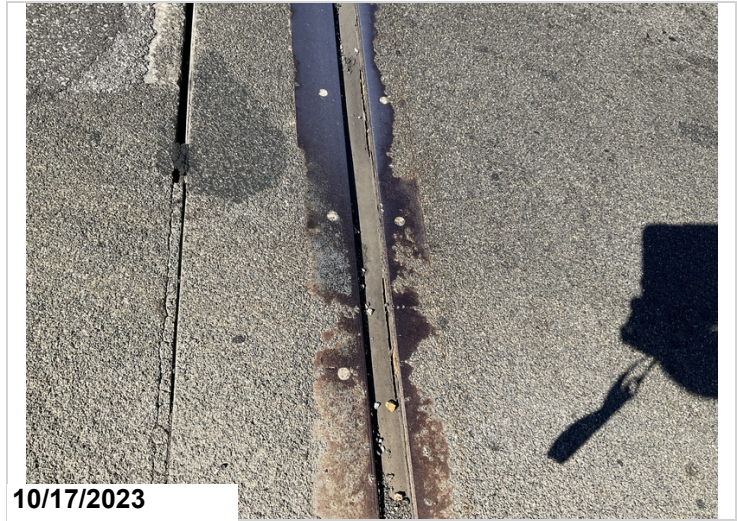
Abutment #2 joint seal has several areas of lost adhesion allowing leakage through joint.
