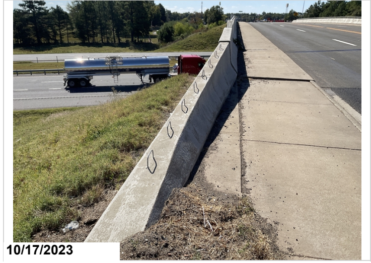
Typical bridge rail end treatment
