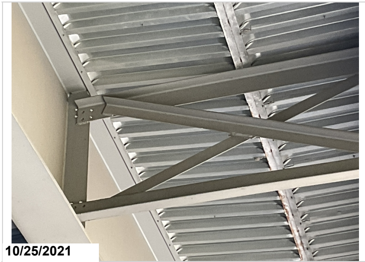
Typical welded rather than bolted diaphragm.
