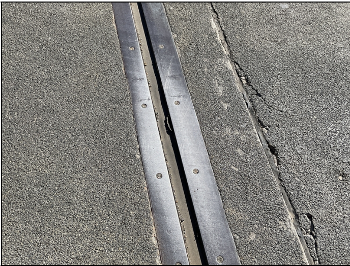
Abutment #2 joint seal right outside lane has one foot of lost adhesion
