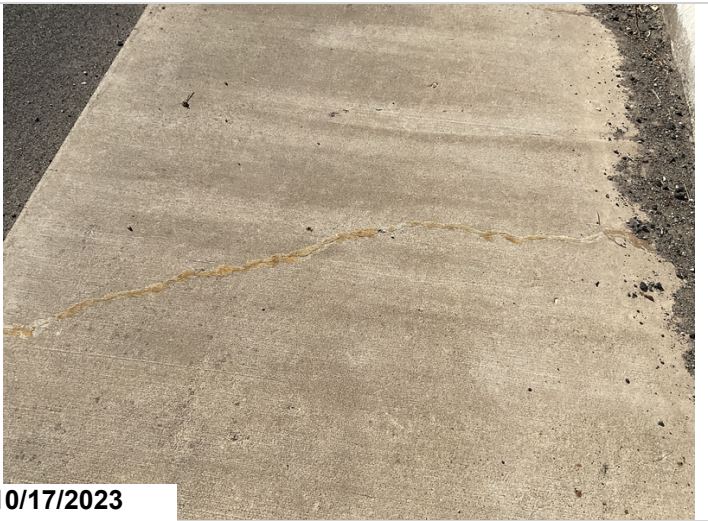
Typical sealed sidewalk crack
