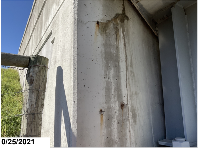
Abutment #2 left end has a few pieces of rebar on surface of concrete exposed, and has horizontal one foot long crack with efflorescence.
