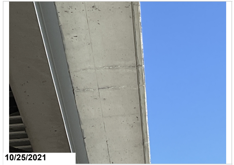
Typical soffit-under surface over hang efflorescence.
