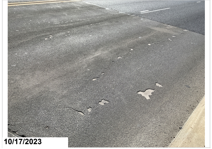
Abutment #2 approach slab right outside lane has several small areas where epoxy overlay is spalled off approximately 20' total affected.
