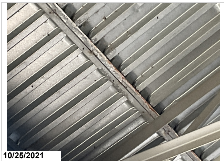
Stay in place forms in center where forms are joined together are starting to corroded.
